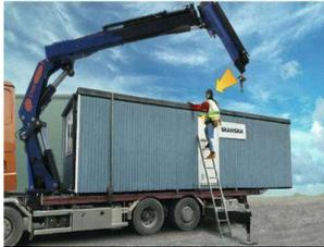
At the storage facility Jens was alone. He parked his vehicle and placed a ladder against the wall of the module. He climbed up to reach the pre-coupled lifting chains on top of the module. Jens was wearing a pair of ear defenders with a built in bluetooth phone connection and was talking on the phone with a colleague and had the crane remote control unit slung over his shoulder.
